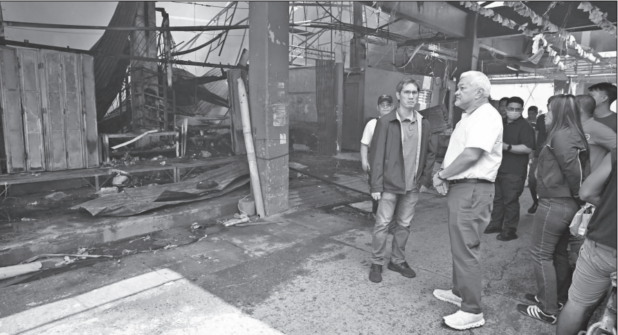
Cong Pogi Lazatin inspecting burned-down sections of the Pampang Public Market.
