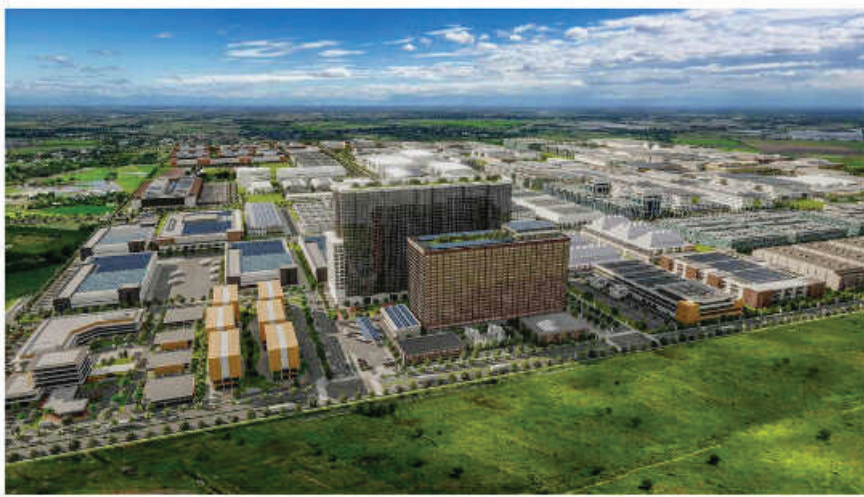
Positioned to anchor Central Luzon's growth as a food manufacturing hub, TARI Estate represents the vision of a future-ready center for advanced and sustainable manufacturing.
