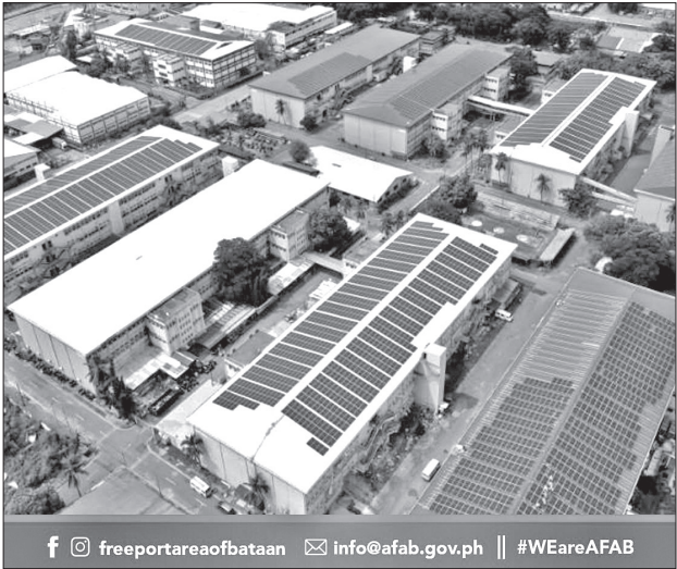
The six-megawatt rooftop solar facility covering 14 factory buildings in the main zone of the Freeport Area of Bataan in Mariveles. PHOTO: AFAB
