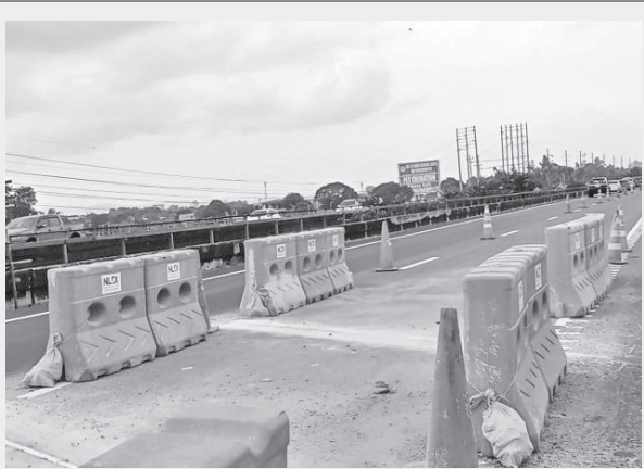
Abacan Bridge along NLEX undergoing rehabilitation. PHOTO: PIA-3
