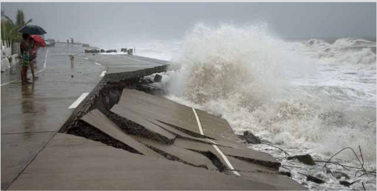
Storm surge destroys a portion of the coastal road at Sitio Tektek, an area identified as a dynamic zone where coastal accretion and erosion occur in cycles. PHOTO COURTESY OF PDRRMO-ZAMBALES
