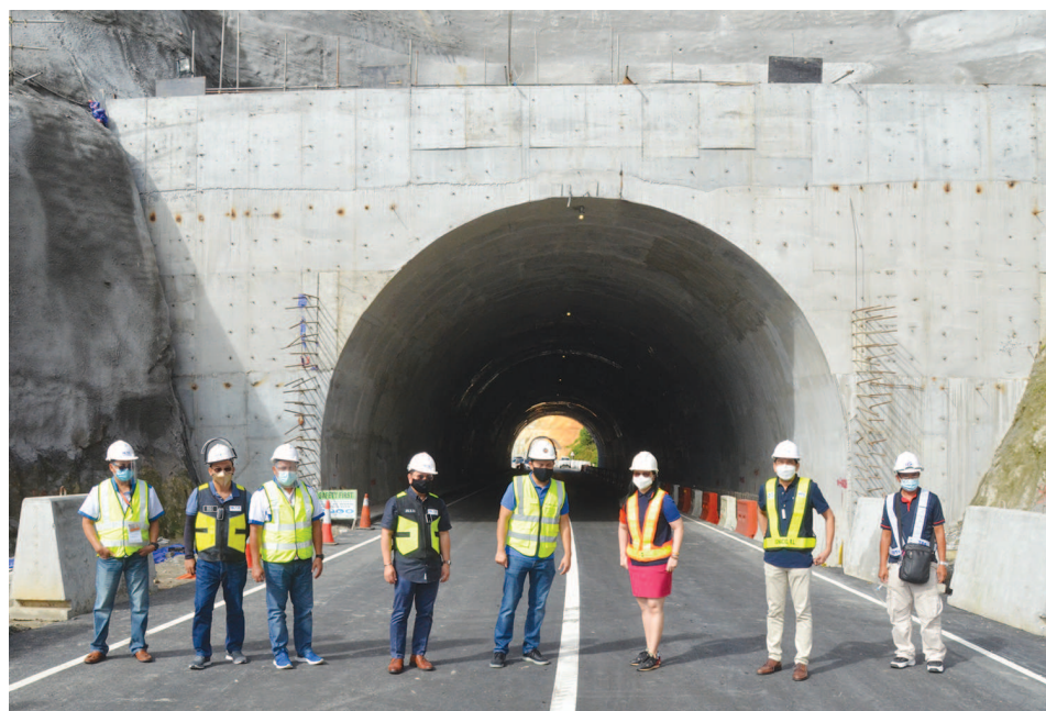
DPWH Secretary Mark A. Villar and other officials pose before the SFEX tunnel. CONTRIBUTED PHOTO
