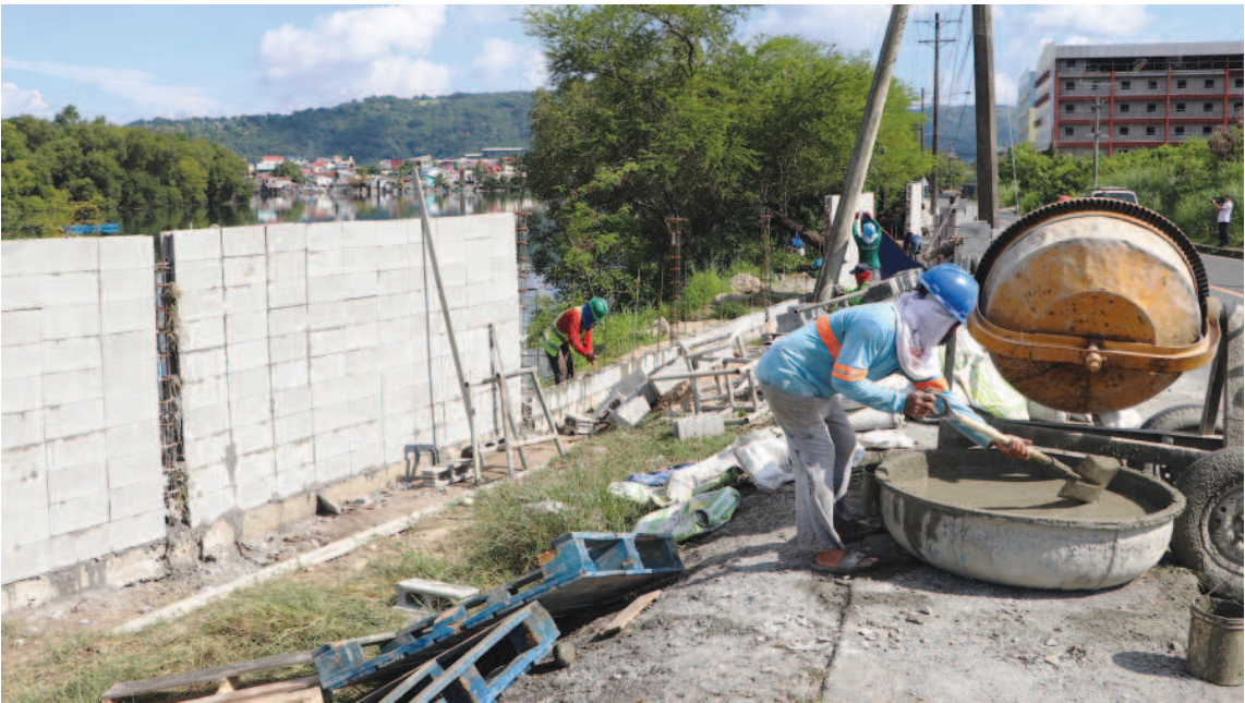
Workers install load-bearing concrete blocks to maximize the integrity of the perimeter fence project at the Subic Bay Freeport Zone. PHOTO BY MALOU DUNGOG
